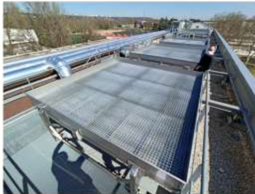
Green Roof - INSA
