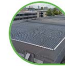
Green ROOF experimental Facility (GROOF)
